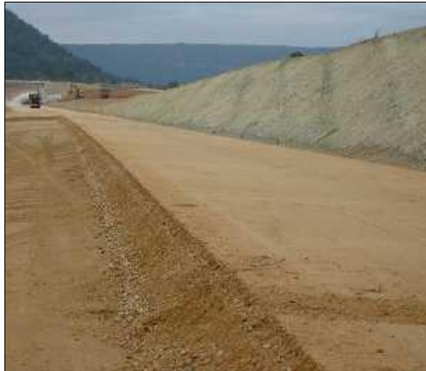
**Figure 1.** *Granular subballast spread*
