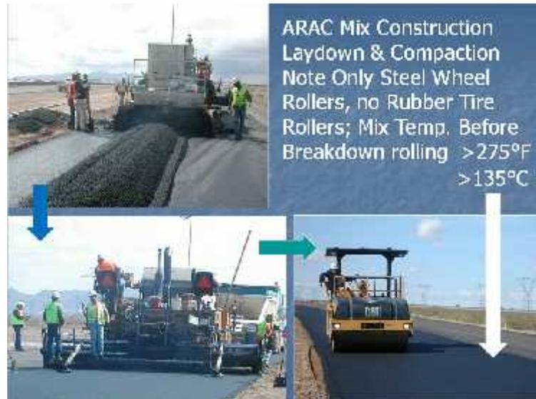
**Figure 16.** Example ARAC Paving with Conventional Equipment
