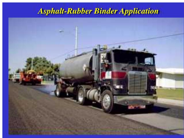
**Figure 5.** *Asphalt-rubber Distributor Truck Applying Stress Absorbing Membrane (SAM)*
