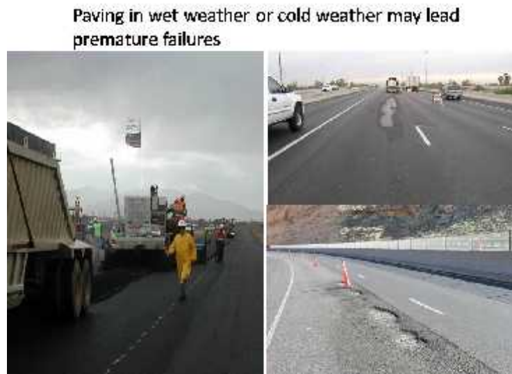
Figure 7. Failures associated with paving in poor weather and/or associated moisture damage
