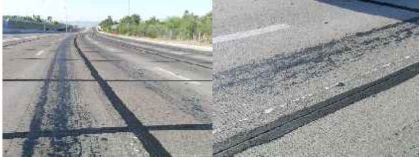
Figure 8. “Track out” caused by hotmix delivery trucks picking up tack coat on their tires at the paving site and depositing the residue on roads off the project as they leave
